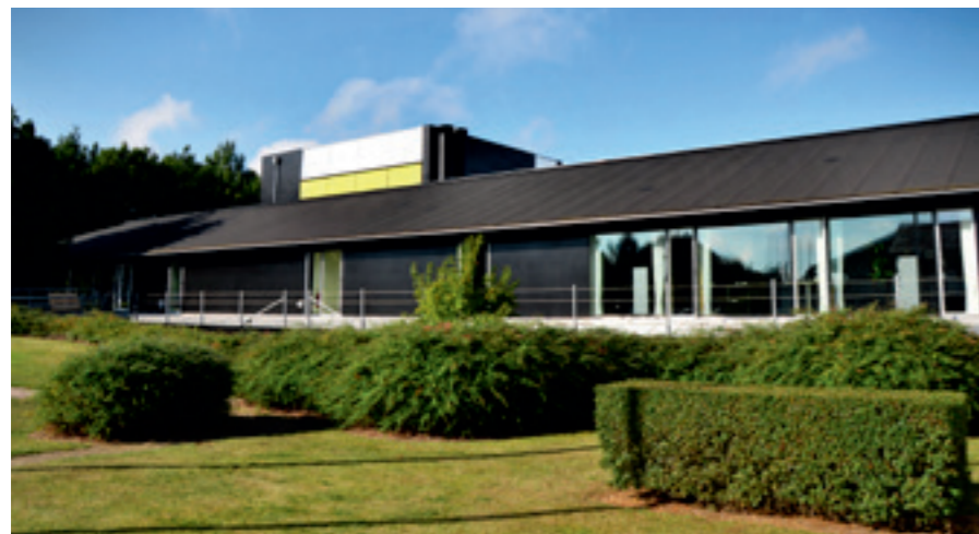
Rockwool International office building was recently renovated to upgrade energy performance. The building envelope was improved with new and better insulated façades and new windows. Also, heat collectors and PV has been installed on the roof for energy production. (Photo: ROCKWOOL)
