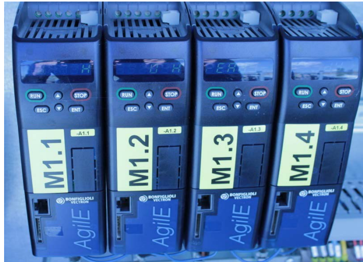
Figure 31A. Frequency converters of the type Bonfiglioli Vectron Agile.
