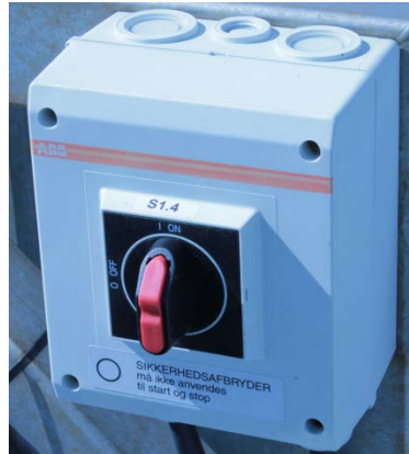
Figure 35A. Manual start and stop button. Located on the lower left part of the frame.
