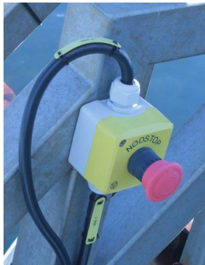
Figure 34A. Emergency stop button. Located on the lower right part of the frame.
