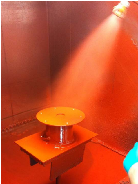
Figure 48A. Top-coat application on disk with airless spray.
