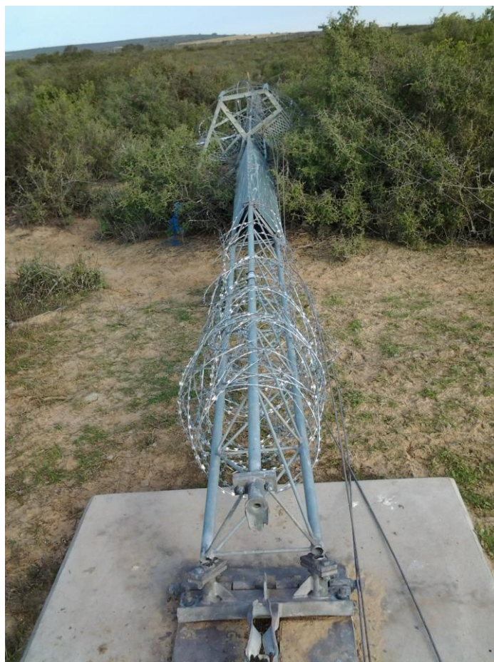
Figure 10. WM04 after the guy wires had been cut by vandals.
