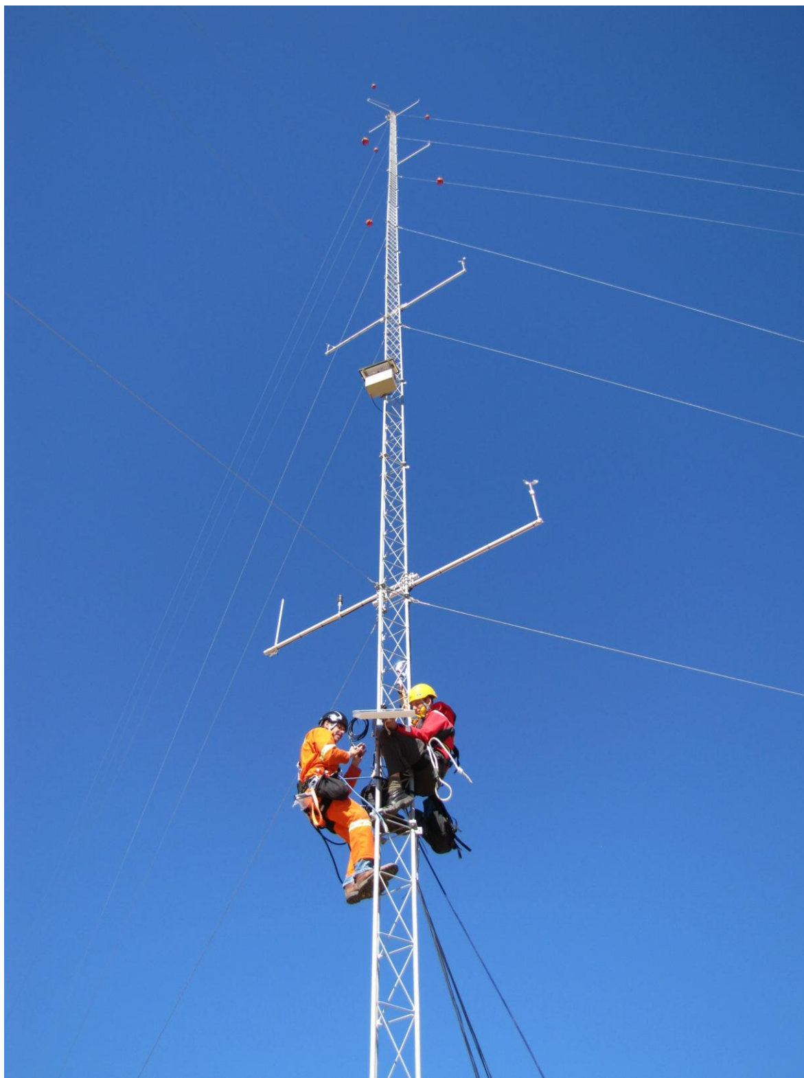
Figure 7. Installing the solar panel powering the data logger
