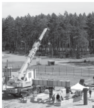
Fig. 2: Pile Test Site at BAM Horstwalde
