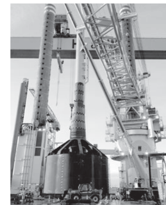
Fig. 1: Full scale bucket foundation on the deck of a jackup vessel
