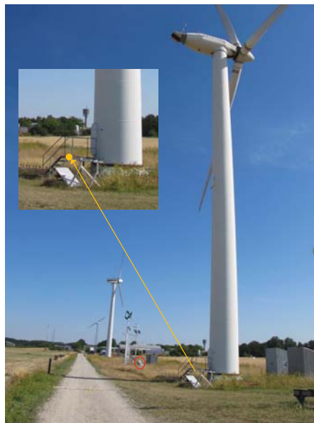
Figure 5: Photo of the NordTank wind turbine used during the measurement campaign. The use point used as a reference for the TST is presented in a zoomed frame. Behind the wind turbine one the short-range WindScanners (R2D1) can be seen.
