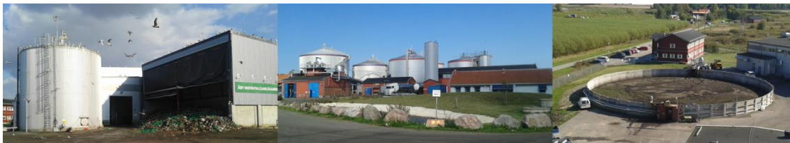
Figure 4. Linköping biogas plant. From left to right: a) Food waste receiving area and pretreatment unit and thermal process tank, b) Main process units including digester tanks and biogas upgrading systems, and c. Digestate storage in open tank.
