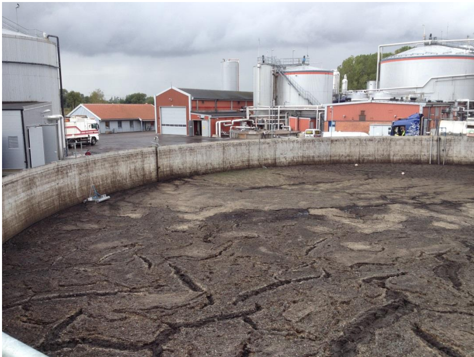
Figure 18. Digestate storage tank and the appearance of the surface layer.
