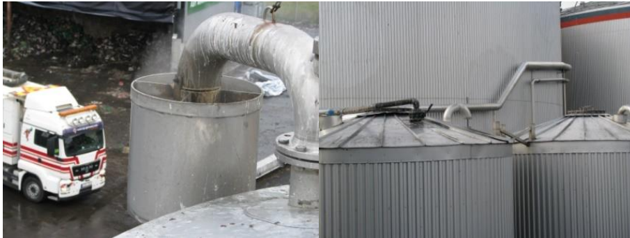
Figure 11 b). Overview of detected leakages, arrows indicate precise location of the leakages (taken from DGC report).
