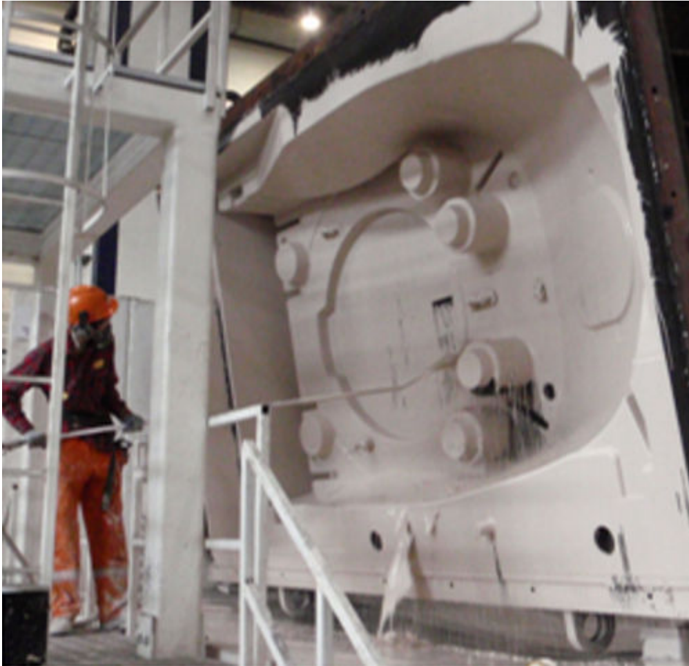
Figure 1.5 Flow coating of large size mould for wind turbine parts production.
