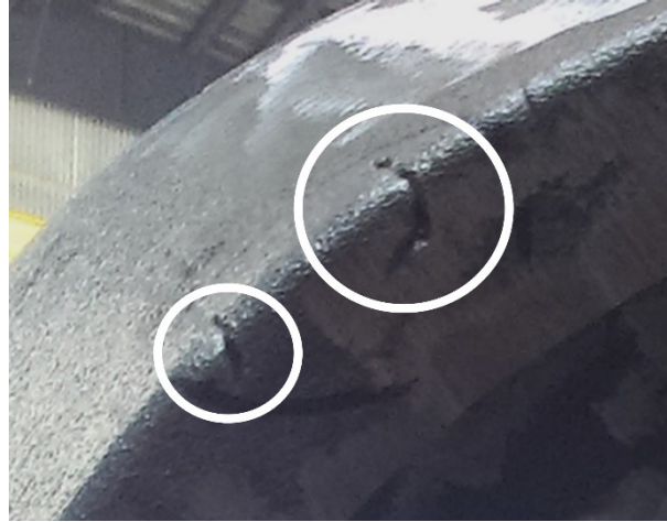
Figure 1. Example of Moisture Related Defect.
