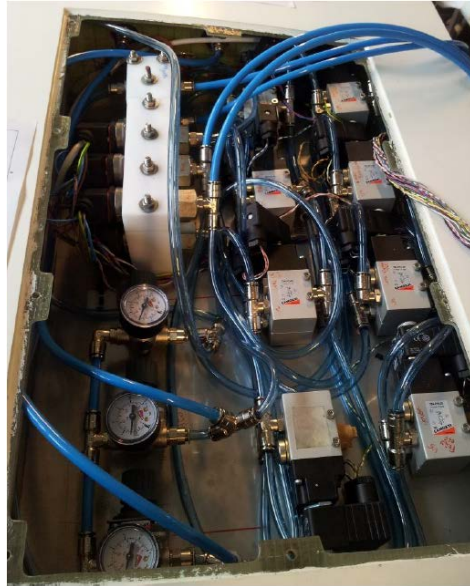
Figure 47 – Pressure switches and transducers implementation in the test section.
