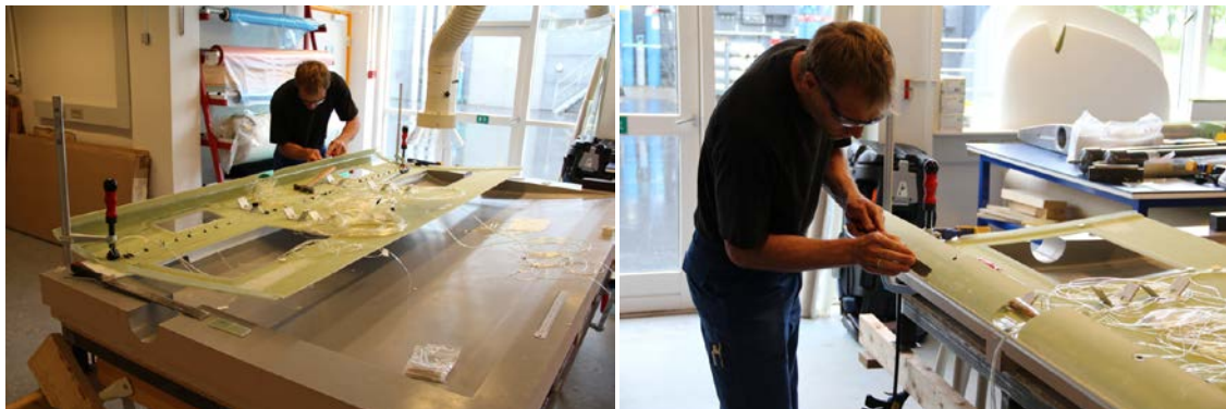
Figure 29 – Left: U-profile overlap mounted at leading edge on the shell structure with hatches. Right: Removal of excess adhesive from the bonding of the leading edge overlap.
