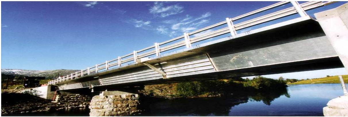
Figure 2: Forsmo Aluminum Bridge in Nordland, Norway (Hydro Aluminium 1996)
