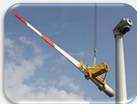
Figur 1: Innovation biography of Blade Dragon, Liftra A/S Blade Dragon is a yoke that enables installing blades on rotors in most angles (+30 to +5). It can perform in wind up to 12 m/s.
