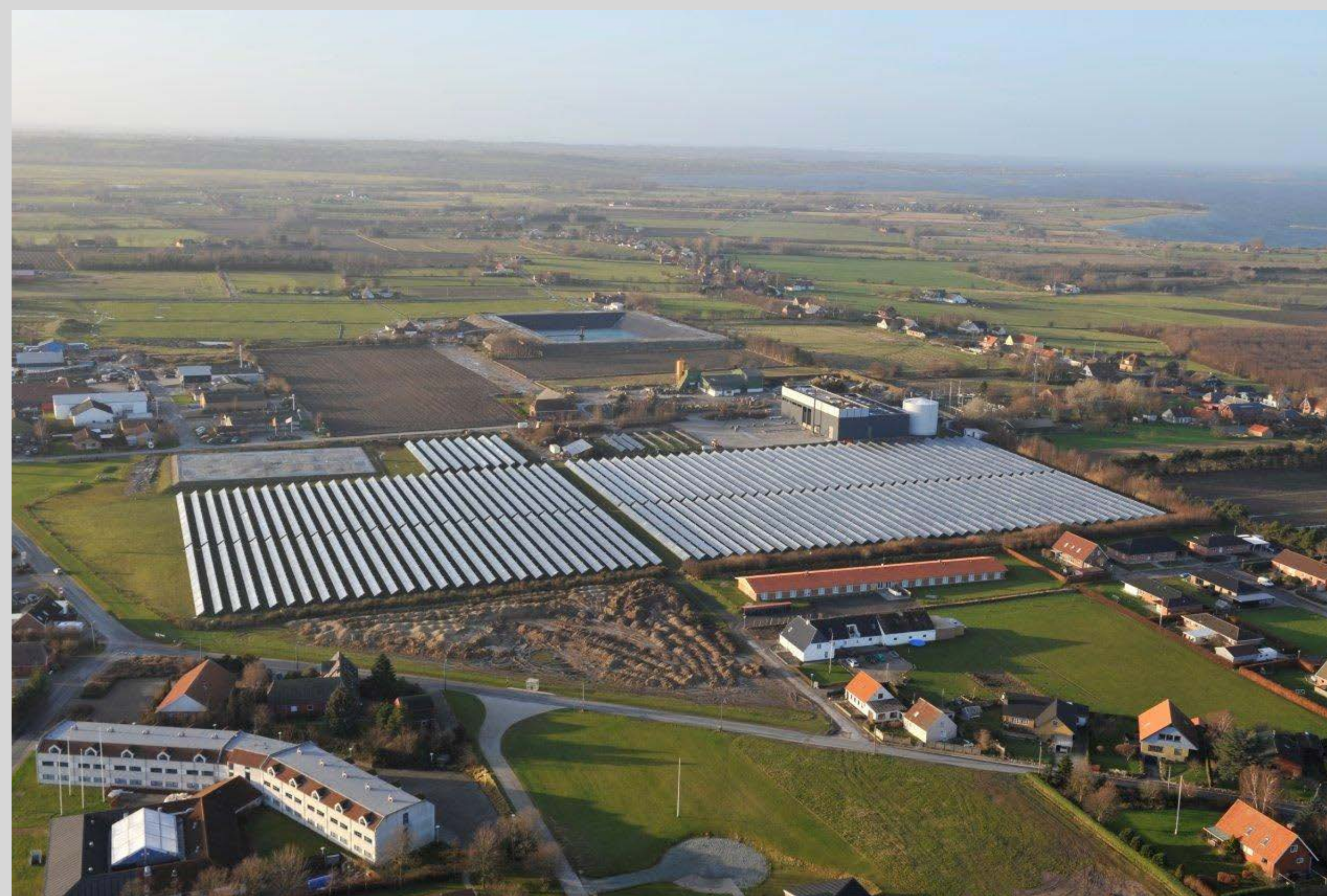
Fig. 5: The plant with storage under construction.
