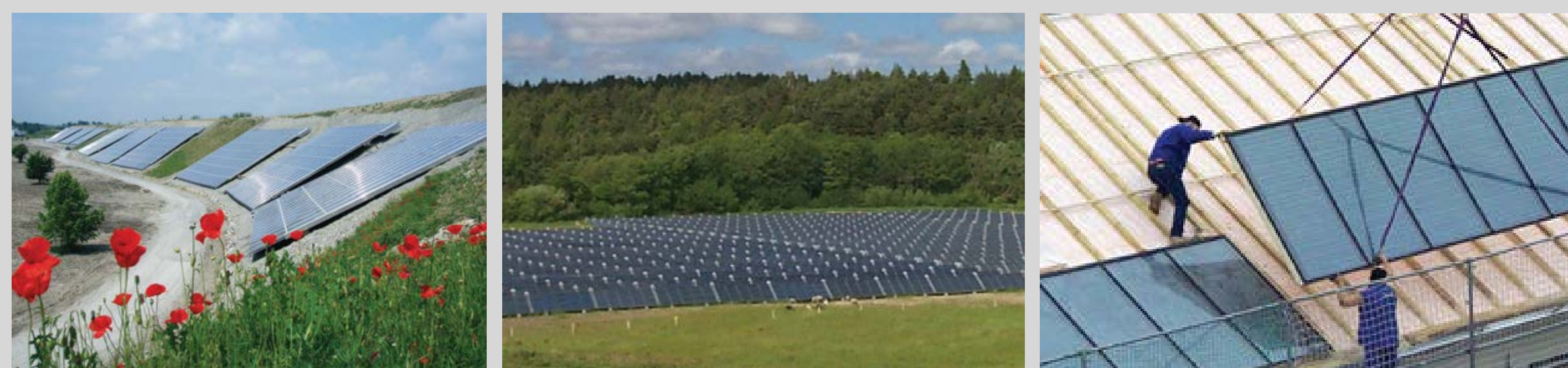
Fig. 4: Examples of solar fields: (a) Terrain mounted, (b) solar field, (c) roof mounted: Source: http://www.solar-district-heating.eu
