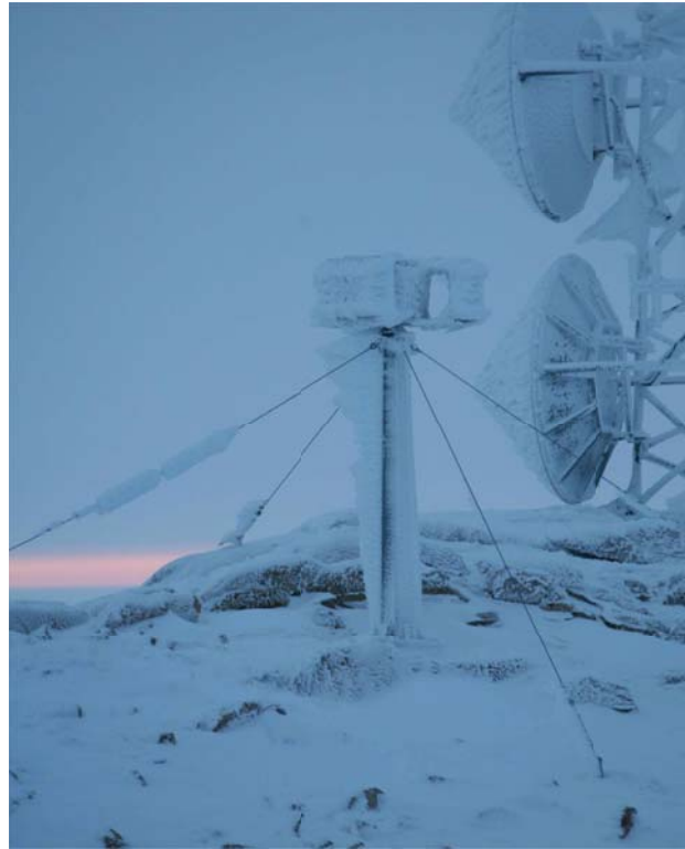
Figure 2.2: A small vertical axis wind turbine located at one of the relay stations in Greenland (photo credit: TELE Greenland).
