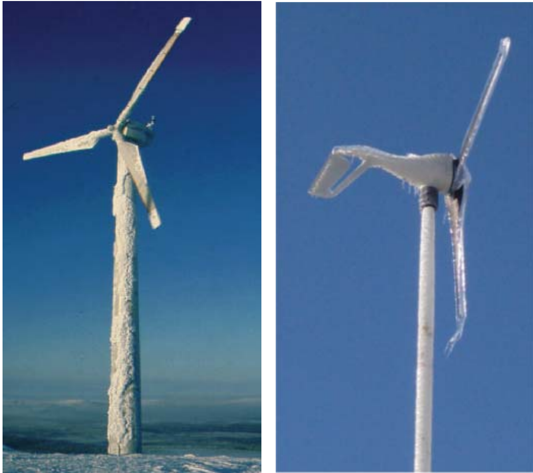
(a) Rime ice accretion on a wind turbine (Tam- (b) Glaze ice accretion on a wind turbine ( http : melin et al. [1998] ).
