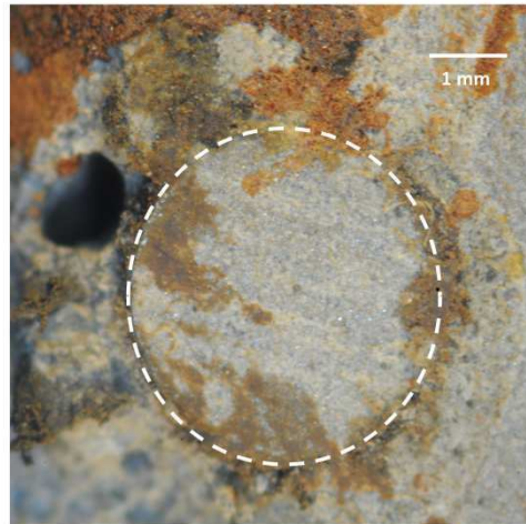
Figure 4.18 Sensor (indicated by broken line) of instrumented rebar located next to main bending crack with signs of corrosion at the sensor and the instrumented rebar for ESE 3 (1.0 vol.% SFRC) beam.
