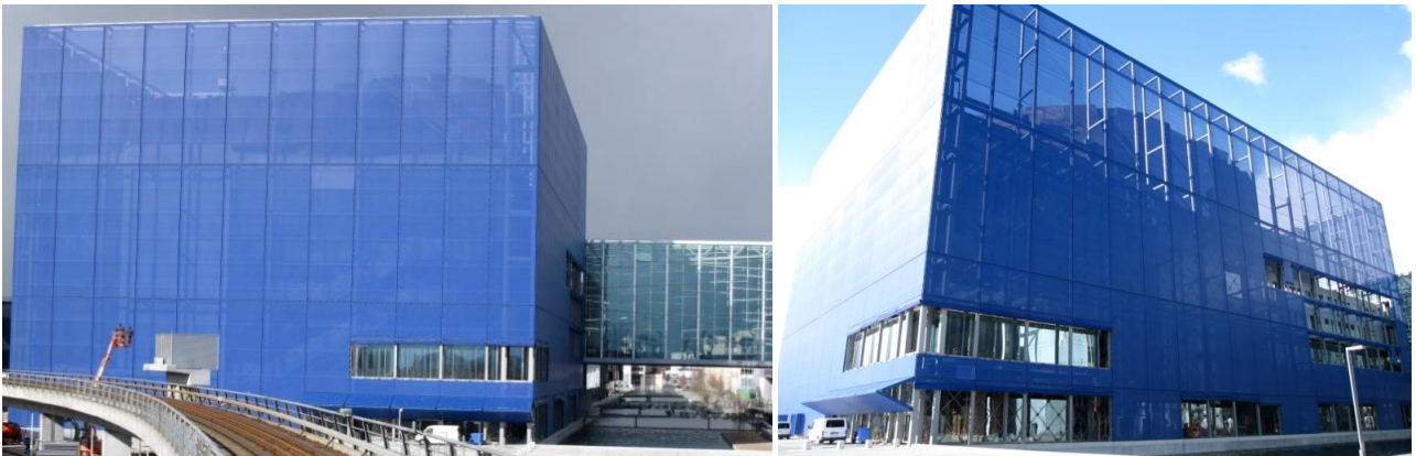
Figure 4 DR Concert House by Jean Nouvel (opened 2009). Left: View from the metro station. Right: View from across the canal. Photographs: © Elisabeth Heimdal.
