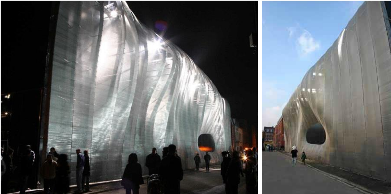
Figure 2 Maison Follies Wazemmes in Lille (2004), France, by architect Lars Spuybroek of NOX. Left: View at night as the textile construction is illuminated from inside, a lighting that can be changed depending on the activities in the building and the time of day. Right: View during daytime. Photographs: © 2009 NOX.
