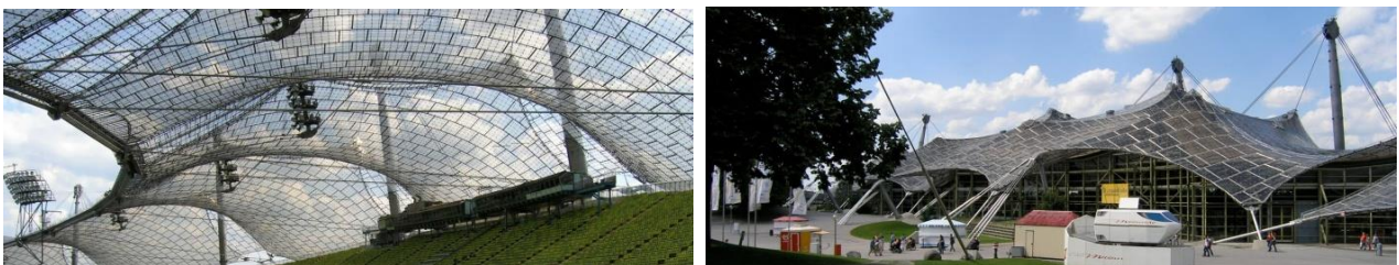
Figure 1 Left: München Stadion by Frei Otto, seen from inside. Right: München Stadion seen from outside. The membrane is covered by glass panels. Photographs: Mistersmed (on Flickr), Limited Rights Reserved.
