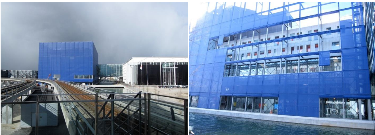
Figure 46 The DR concert hall. Left: Seen from the metro station during daytime. Under the cube covered by the blue textile, one can barely see the underlying building with a different shape. Right: One of the sides of the cube close-up. The different modules of blue textile can be rolled up. Photographs: © Elisabeth Heimdal.
