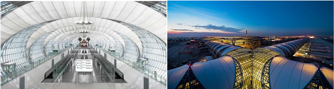
Figure 8 Suvarnabhumi International Airport Bangkok by architect Murphy/Jahn (opened in 2006). Left: One of the terminal buildings seen from the inside. The building envelope is partly made of glass and steel, partly of the three layer membrane system. Right: Airport seen from the outside. Photographs: © Jahn.
