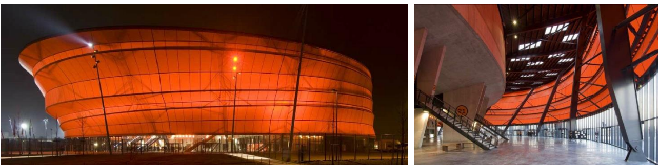
Figure 3 Zénith Concert Hall in Strasbourg, France (opened in 2008). Left: View from outside. Right: Lobby of concert hall. Photographs: © Massimiliano Fuksas.
