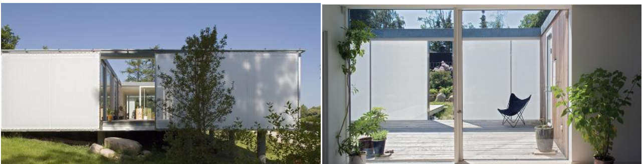
Figure 5 Summerhouse in Jørlunde, Denmark, by Dorte Mandrup Architects (2004). Left: View of the house from outside. The white screens are made of metal frames onto which textiles have been stretched. The frames are movable and provide shade and privacy to the terrace. Right: View of the terraces from the inside of the house. Photograph: © Dorte Mandrup.
