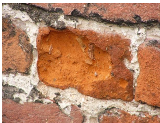
Masonry. Picture: Lisbeth M. Ottosen (2007)
