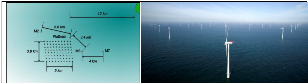
Figure 51 The Horns Reef 1 wind farm layout of 80 Vestas V80 wind turbines
