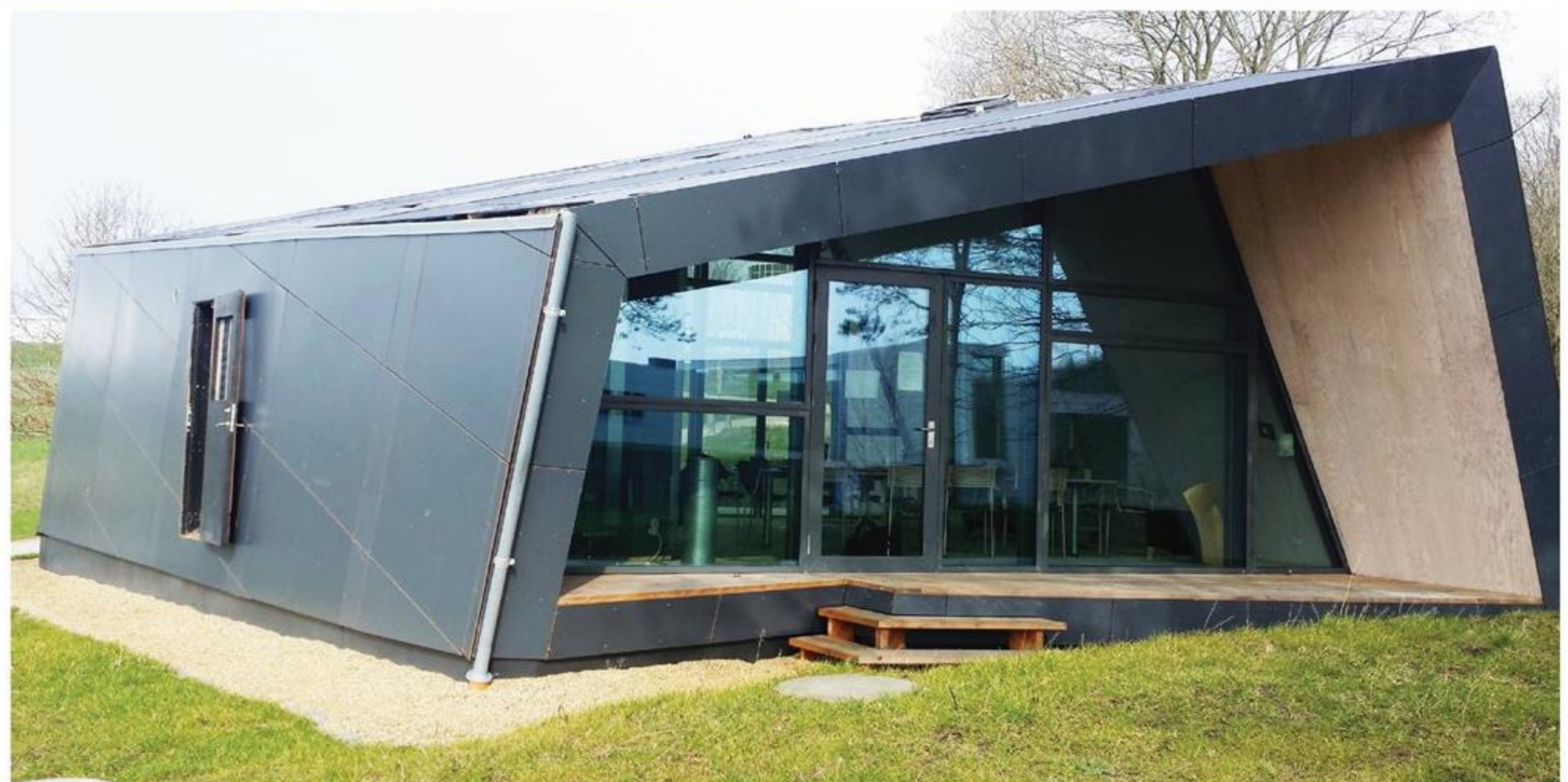
Figure 1: The South façade (top) and the North façade (bottom).
