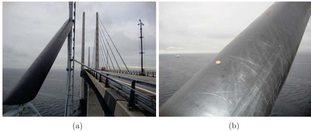
Figure 3.4: Deck level cable section at the Øresund bridge (a) and evidence of local alterations of surface roughness (b).
