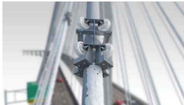
Figure 2.22: Custom-designed ice/snow sweepers to be fitted to the stays at the Portmann Bridge in Vancouver, British Columbia. (Pictures from http://www.news1130.com/ ).
