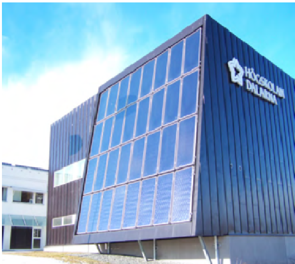
Figure 2. Building integrated collector field for the studied district heat augmented solar heating system at Högskolan Dalarna.
