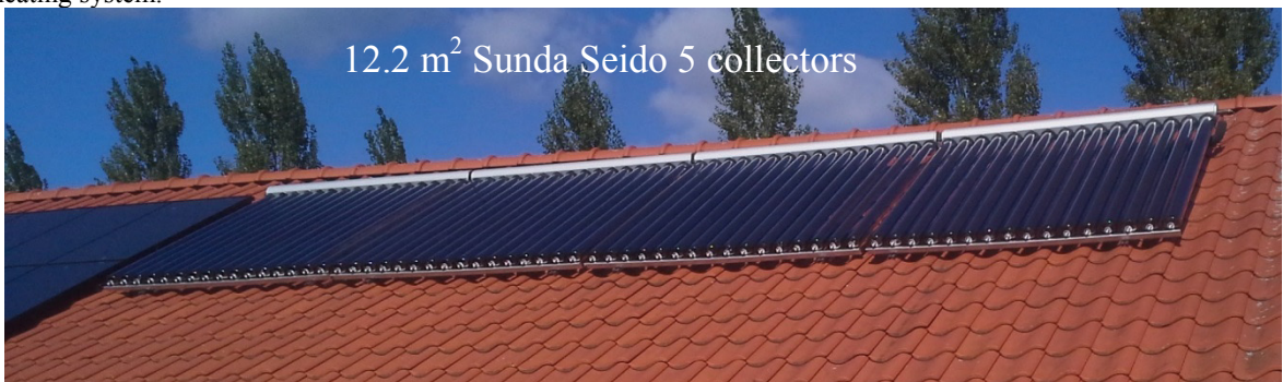
Fig. 4. Sunda Seido 5, Vacuum tube solar collectors, in the demo system . (The PV system to the far left only interacts with the electric grid.)
