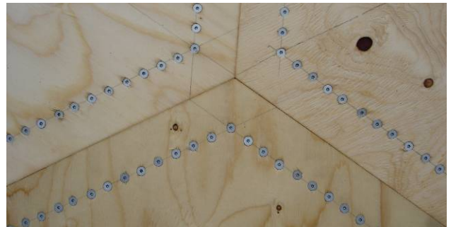
Fig. 10. Detail of the screwed connection between elements.
