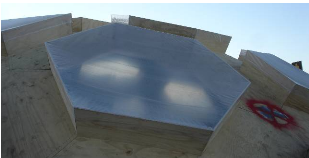
Fig. 15. Opening covered with plastic film.
