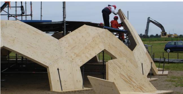
Fig. 19. Assembly of the 2012 dome.
