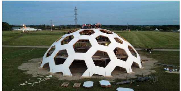
Fig. 21. Shell structure completed.
