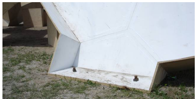
Fig. 23. Edge element anchored with tent stakes.
