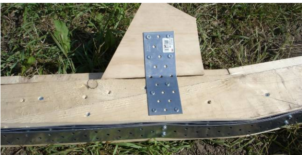
Fig. 6. Ring beam detail before elements are mounted.
