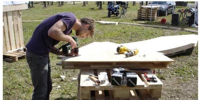
Fig. 9. Preassembly of connection plates on an edge element.
