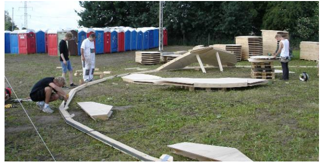
Fig. 8. Ring beam under construction.
