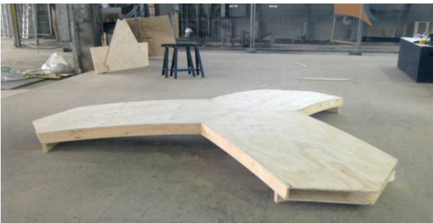
Fig. 5. Test assembling of the first three prefabricated elements.
