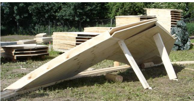
Fig. 7. Ring beam with two edge elements. At the top between the elements the connection plates are seen.
