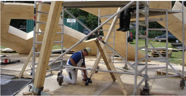
Fig. 17. Manipulation of shell surface by hydraulic jacks in 2011.
