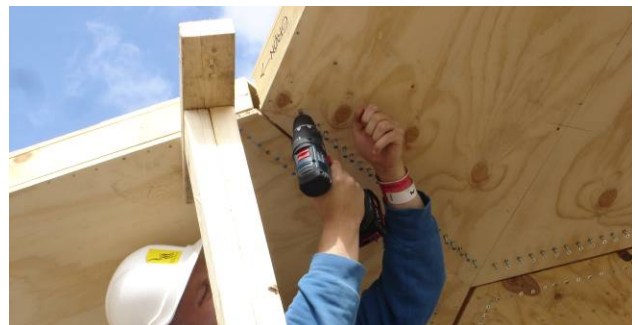
Fig. 11. The last element in place.
