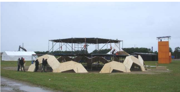
Fig. 18. Scaffolding for the 2012 dome.
