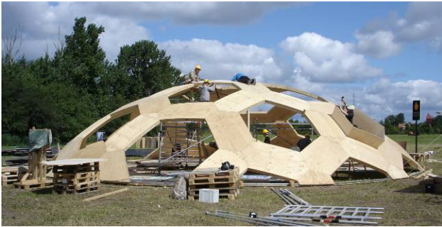
Fig. 12. Completion of shell structure before side panels is added.
