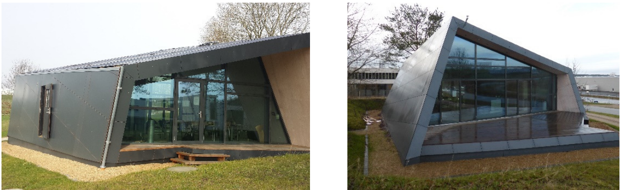
Figure 1 –The South façade (left) and the North façade (right)
