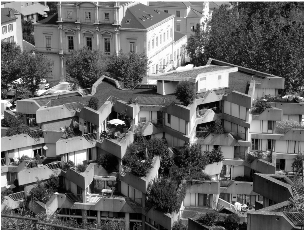
Figure 5-5 Diversity in building form, Jean Renaudie, La Cité des Étoiles, Givors, France (1974–1981), 270 dwellings, shops, library, theatre, and police station. Photograph by Louiseau (2013).
