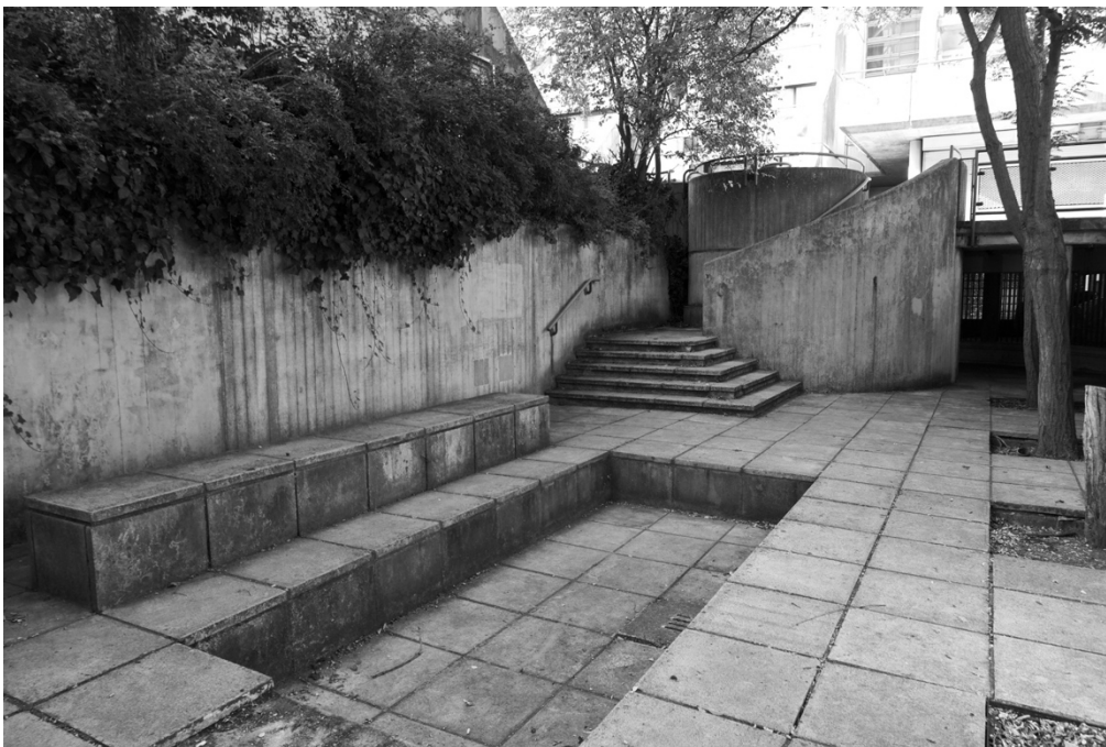
Figure 5-12 Distinct and intimate space for gathering or solitude, which adjoins block A and B with block C; Neave Brown, Alexandra Road (1968-1979), Camden Council, London Borough of Camden.
