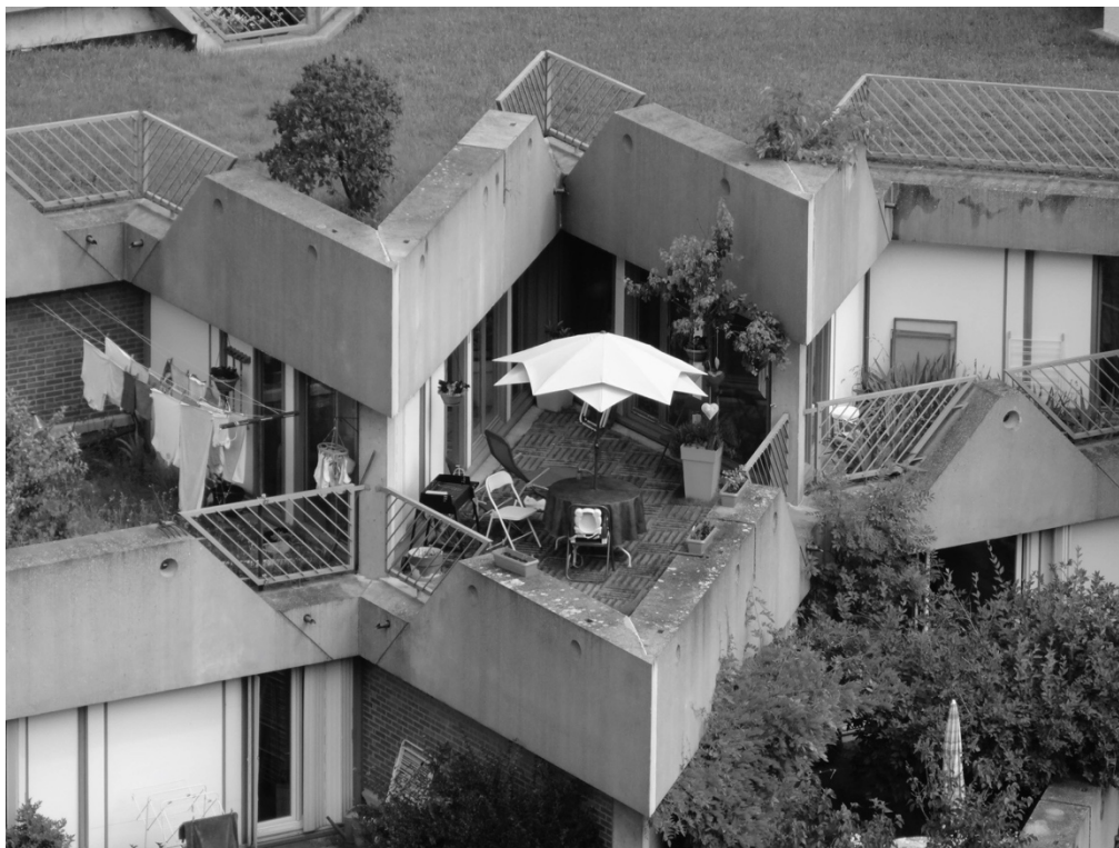
Figure 5-14 View of private terrace, Jean Renaudie, La Cité des Étoiles, Givors. Photograph by Louseau (2013).
