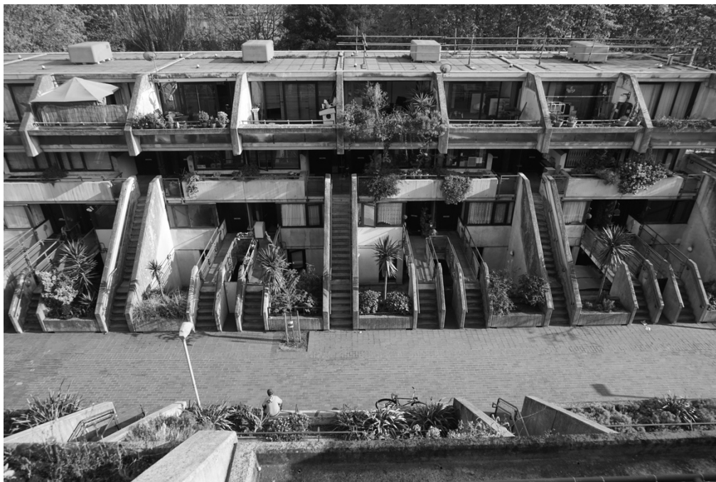
Figure 5-8 Block B, system of staircases that connect the pedestrian street to the front door of the upper level units, seen from high-level walkway on block A; Neave Brown, Alexandra Road, Camden Council, London Borough of Camden. Photo by ACME London (2019).
