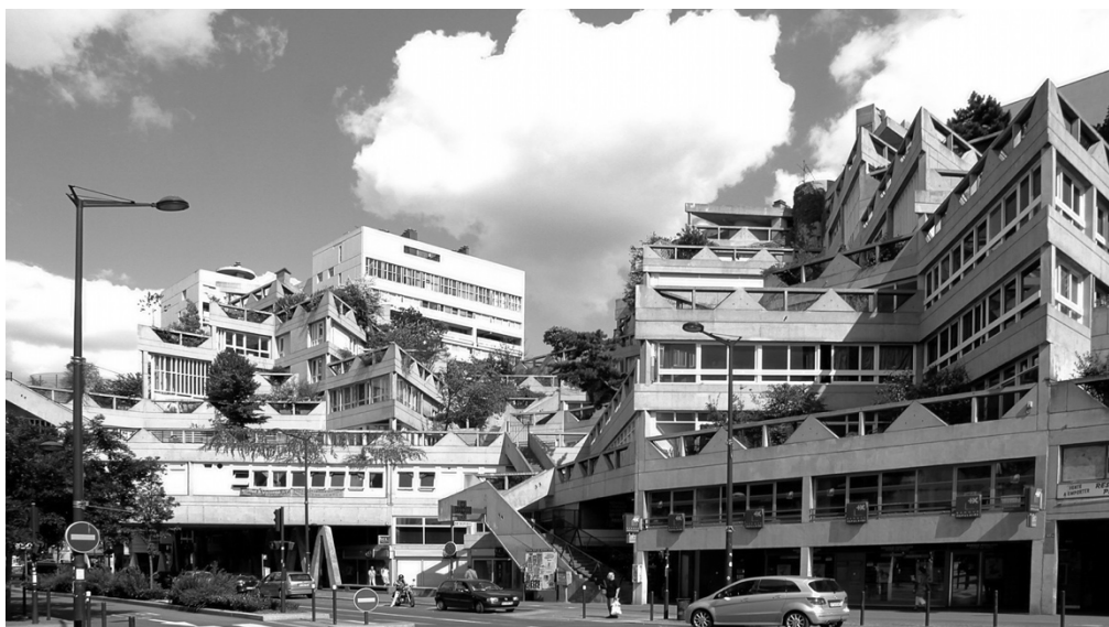
Figure 5-4 The Jeanne Hachette Complex, Jean Renaudie, Ivry-sur-Seine, Paris (1970–1975); 40 dwellings, cinemas, retail, office, and parking. Photograph by Valette (2013).
