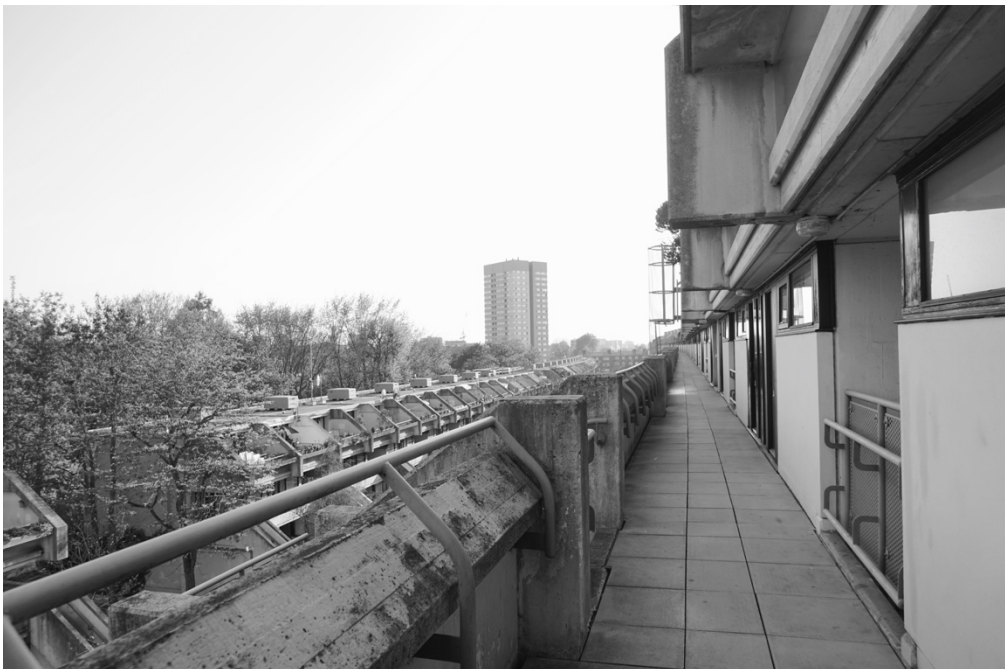
Figure 5-9 View from the high-level walkway on block A, right , overlooking block B, left , with the tower of Hampstead’s Abbey estate in the background; Neave Brown, Alexandra Road, Camden Council, London Borough of Camden. Photo by ACME London (2019).
