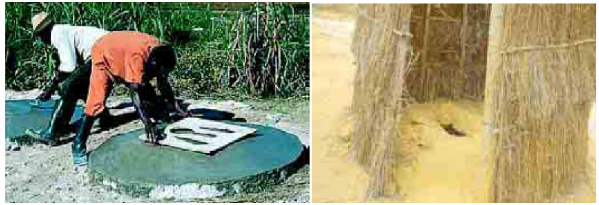
Fig 1: Real slabs constructions for latrines 41 . Fig 2. Some traditional latrines in Nampula illustrating sanitation problems in the neighbourhood.
