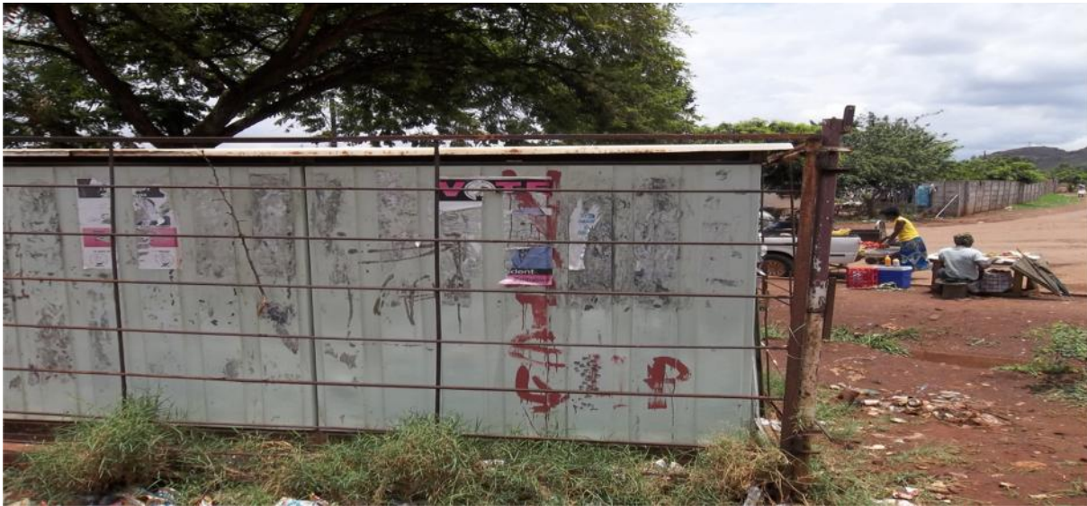
Figure 4.3 Graffiti inscribed on an electricity sub-station
