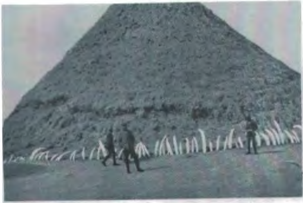
PICTURE 11: The distant and close-up pictures of the pyramid of Ngundeng, the 19th-century king of the Nuer. The Nuer country is hardly 200 Kilometres north of the Kenya-Sudan boundary. The pyramid is thought to have been initiated by Ngundeng around 1900 AD and completed by his son Gwek. This pyramid is called Deng Kur and is the biggest in the Nuer country. Constructed of baked earth and ashes, it was estimated by the pioneering European colonial officers to be 50 feet high and 300 feet in
