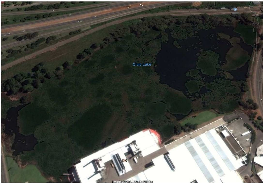
Figure 4.2: Area covered by water hyacinth in the Civic Lake (Satellite imagery of March 2010)
