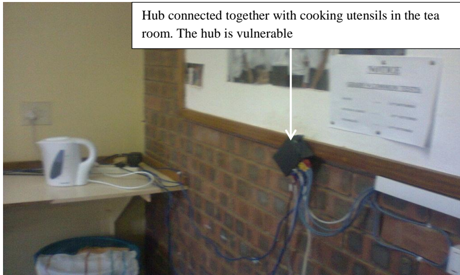
Figure 7.6a: Switch connected together with water mugs in the tea room
