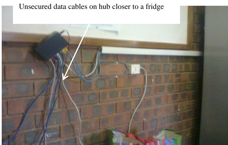
Figure 7.6b: Network hub closer to a refrigerator in tea room
