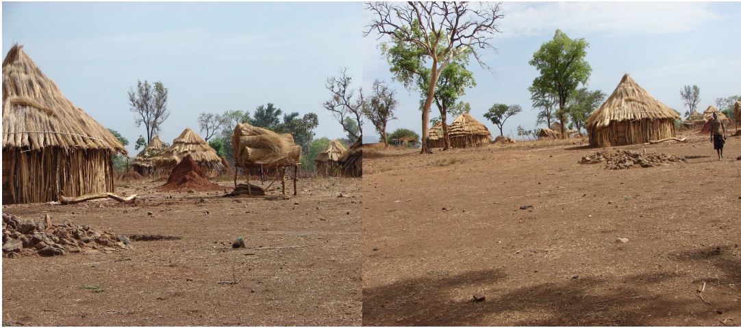
Figure 6. 8. Villagization, Typical Thatched-Roof House under Construction, 2011
