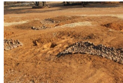
The preparation of the planting of indigenous trees at the MPC, using stones as well as the gradient, the runoff of the rainwater is maximised to ensure that trees are watered. The area around the tree bark will be used to plant seedlings which can also maximise the rain water run-off and thus reduce the labour in terms of watering of seedlings.
