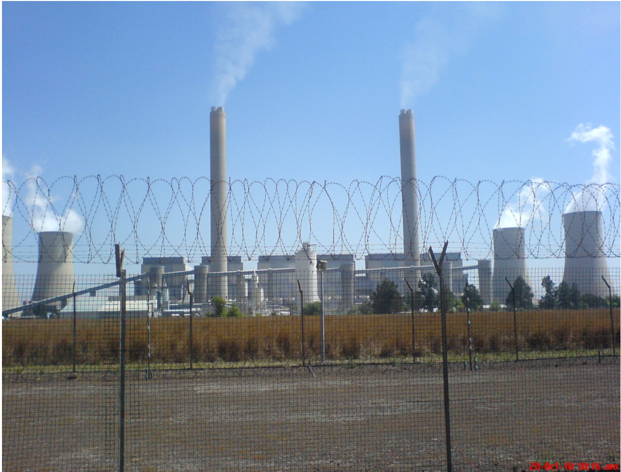
. Picture of power plant showing two stacks where emission is released and four coolants
