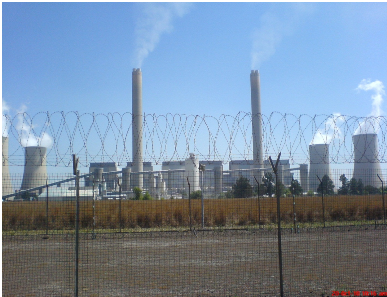
Fig 3.1. Picture of power plant showing two stacks where emission is released and four coolants
