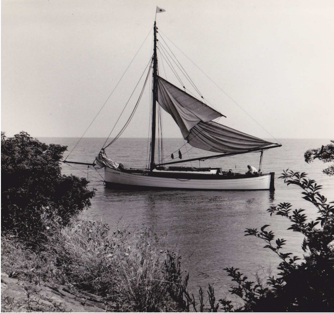
Figure 3-14: Loose brailings on a gaff-rigged sail (Photo: Henny Buddingh, private collection).
