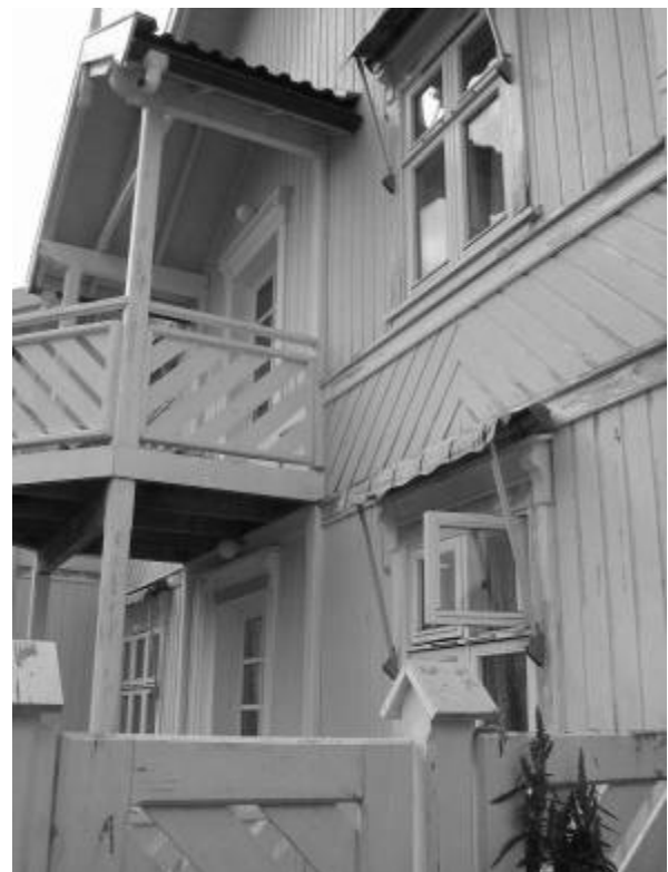
Figure 4.9. This collection of three images (one on the next page) of porches, plantings, awnings, complex windows and roof lines shows how elaborate the edge between indoors and outdoors can be. People who dwell within such architecture have a high degree of choice and control over their daily and yearly connection to nature in a relatively little space.
