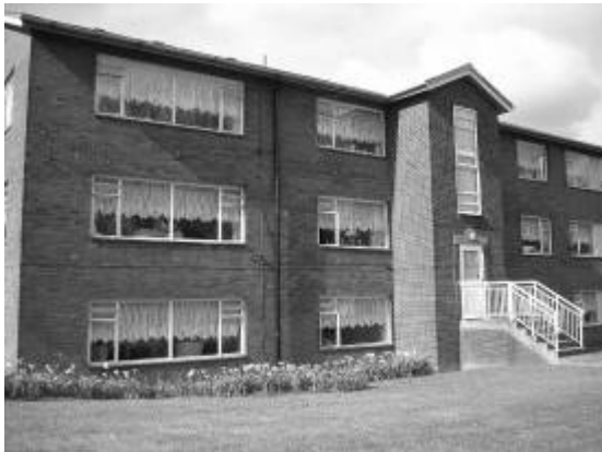
a) Addition of a protected fire stairwell
