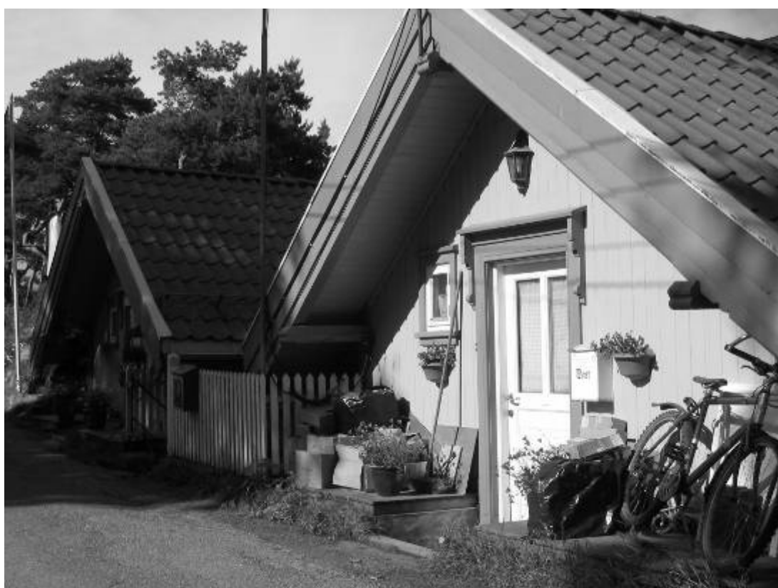
Figure 4.10. This house in Langesund, Porsgrun Commune, Norway is two storeys with a ground floor entrance on both storeys owing to its position on the steep slope overlooking the fjord. This arrangement was mentioned in section 4.3.2.3 and shown with Figure 4.1 as a way to utilise a slope to afford a person architectural outdoor access, avoiding confinement to an upper floor for a person with dementia.
