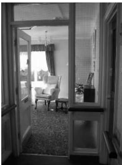
c) door & partition close off air flow from adjacent areas
