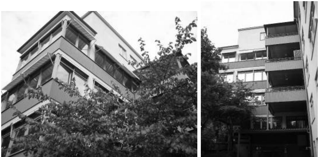
Figure 4.11. This building contains flats for older people provided by social services in the Sabbatsberg area of Stockholm, Sweden. The adjustable striped awnings and large openable windows on three sides of a common room are situated directly adjacent open-air porches (pictured on the right) on all floors.
