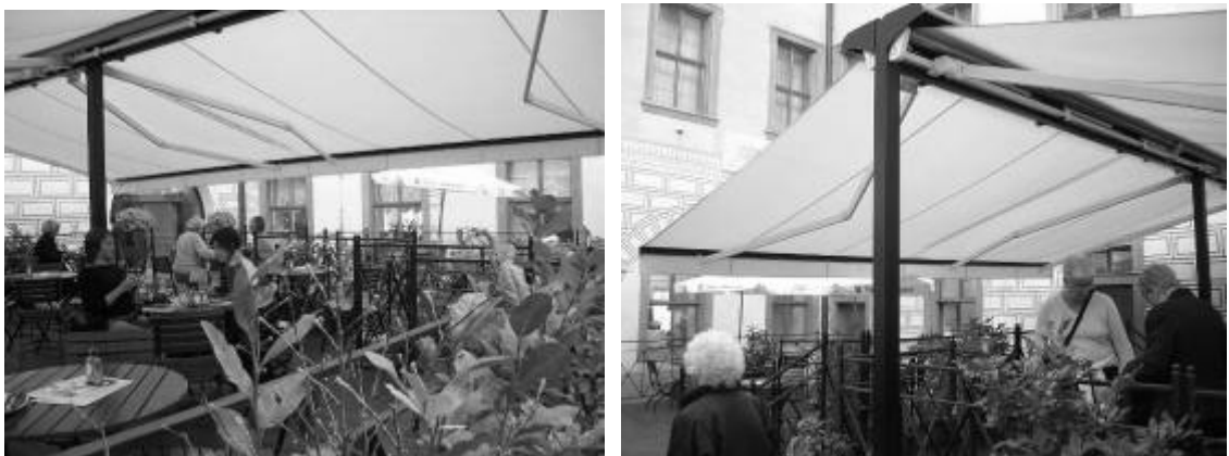
Figure 4.8. This example shows the transformation of space made possible by membrane structures when used to create a sheltered, heated year-round outdoor dining area in the central courtyard of a building.
