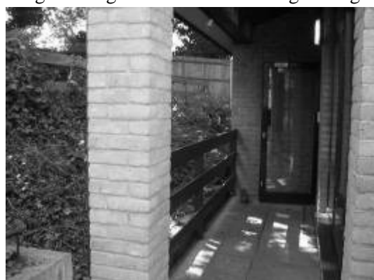
Open door & handrail to large lounge
