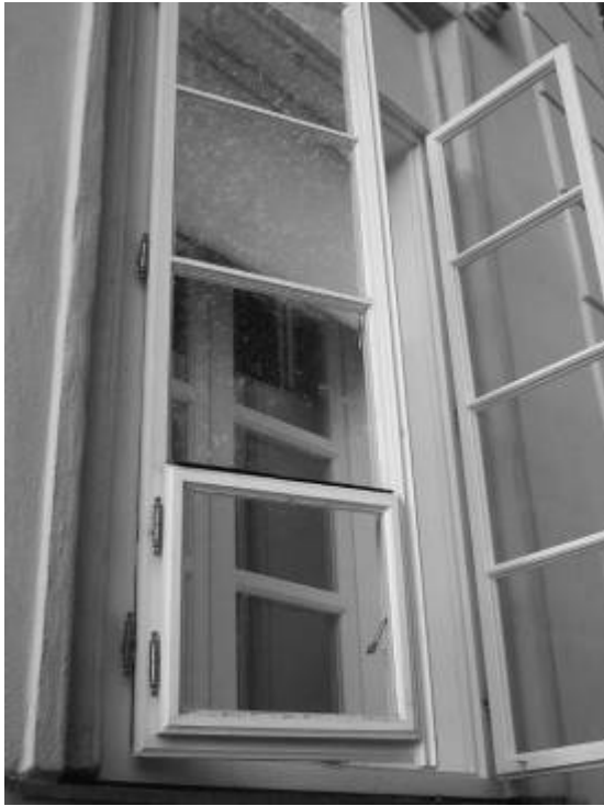
Figure 4.7. The complexity of this window set affords unlimited possibilities to the resident to modify the temperature, breeze, sounds and sun entering the home. It also provides space between the two sets of windows for growing plants and displaying ornaments. Notice the pull-down shade hanging between the inner and outer windows as well as the lowest square pane which is openable.
