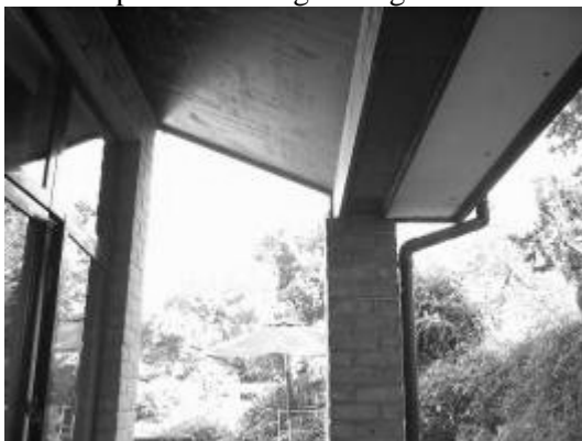
Roof structure over walkway to large lounge
