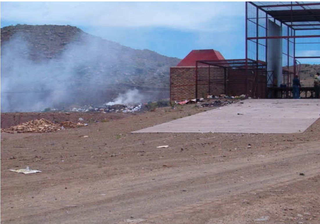
Figure 4-3. The incinerator that was installed at a landfill site in the Maletswai area in 2003 and was not operational at the time of follow-up a year later (note missing chimney). Waste was instead being burned on site.
