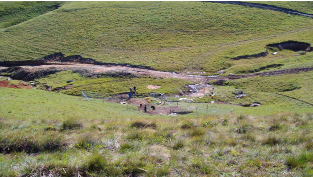
Figure 3-20. Example of a high impact and default project (water supply scheme) in the Engcobo Municipal area 9 .
