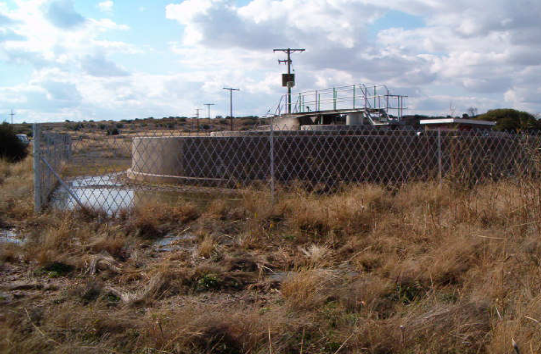
Figure 4-2. A sewage treatment package plant constructed in 2002 that two years later no longer functioned optimally as indicated by the ponding of effluent on site.
