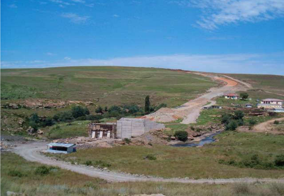
Figure 3-1. Road and bridge in the Elundini area during the construction stage.
