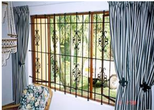
Picture 20: Example of burglar proofing on the secure (inside) side of the window frame
