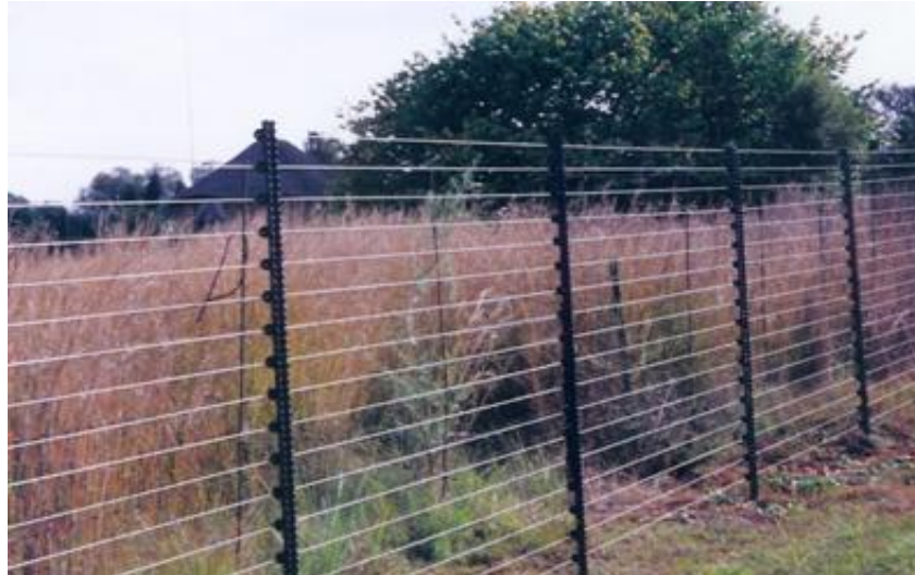
Picture 7: Example of electrified fencing as the perimeter
