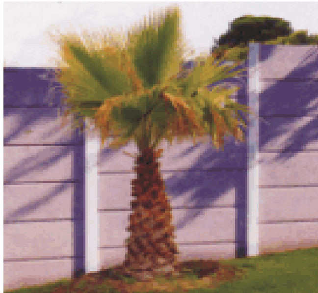
Picture 3: Example of a pre-cast cement slab walling
