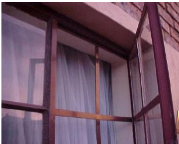
Picture 19: Example of burglar proofing integrated with the window frame
