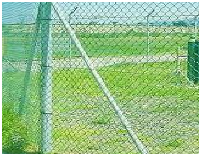
Picture 4: Example of a diamond mesh wire fence partition
