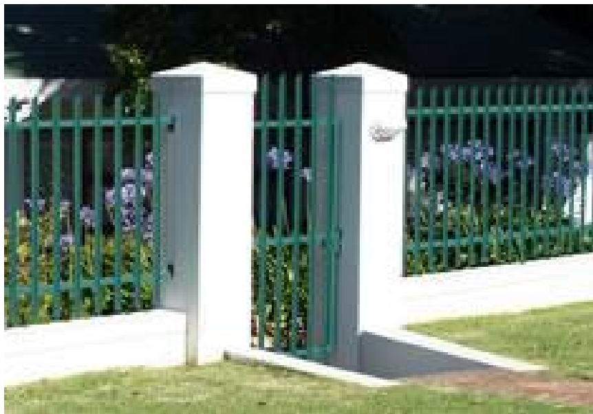
Picture 11: Example of stand alone pedestrian gate
