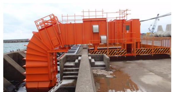
Photo.3 Wave power generation facility completed (Jan.2015)
