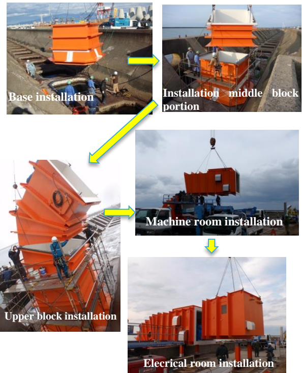
Photo.2 Power generation facility under installation (Dec.2014)
