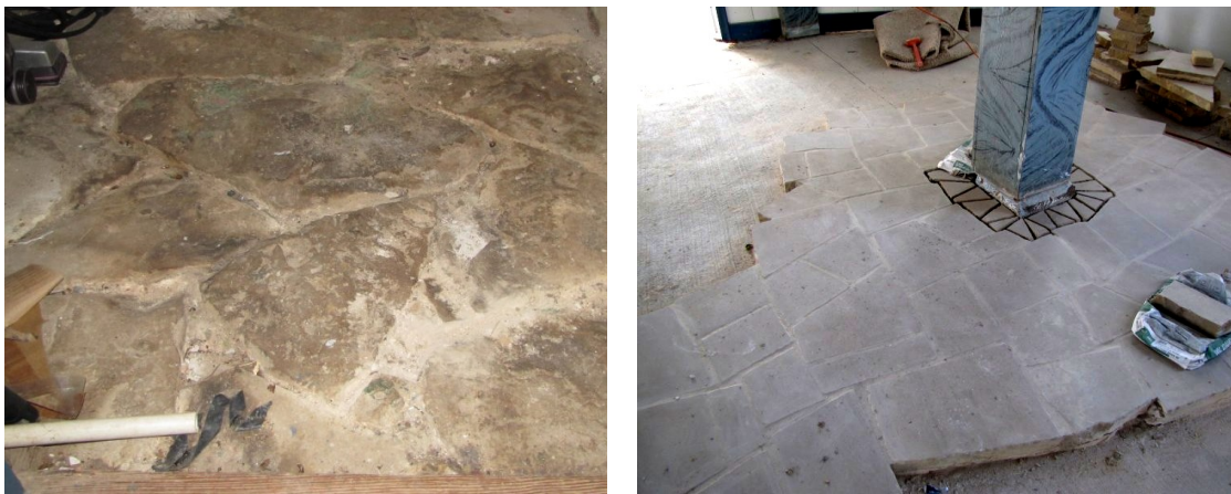
Figure 4-8. Original stone floor (left, St. Paul Lutheran 2010) and new stone floor (right, St. Paul Lutheran 2010)
