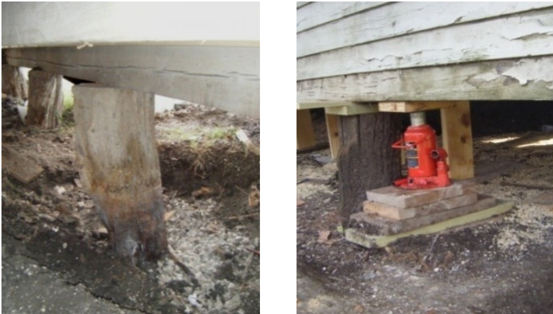
Figure 3-3. Original foundations (left) and jacks used to level structure (right)
