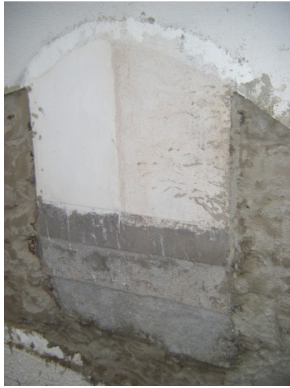
Figure 4-6. Four stages of plaster repair
