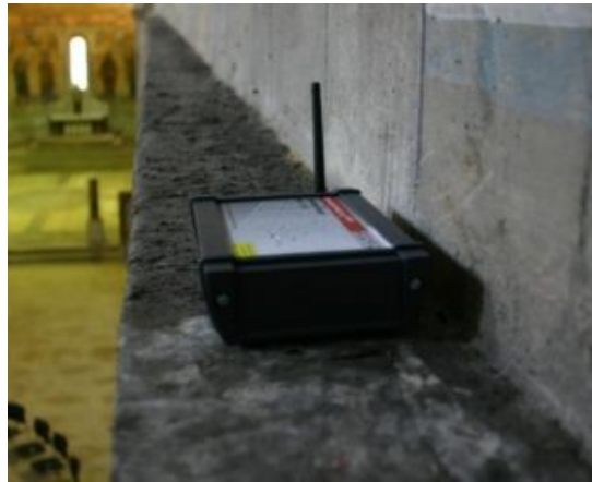
Figure 5-4. Wireless sensor installed in the Johanniskirche (SmartMote 2010)
