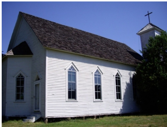
Figure 3-1. Exterior view of Frankford Church
