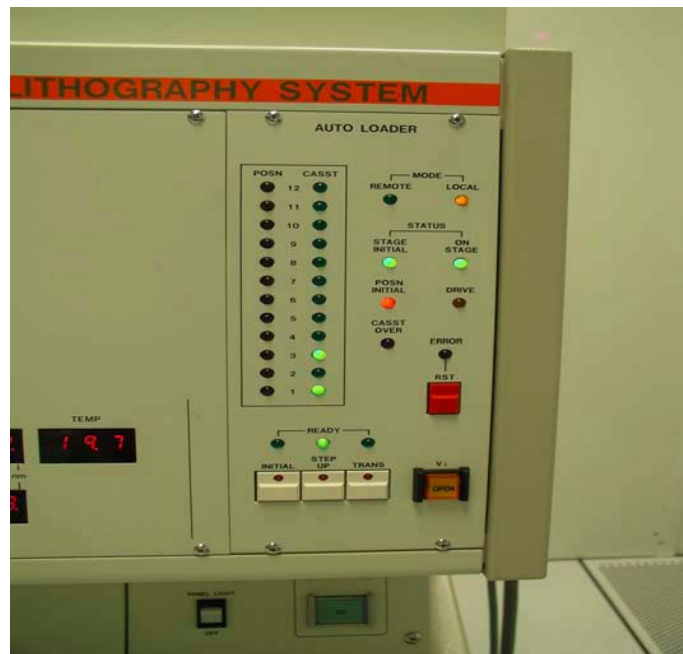
Fig. 71. Auto loader (wafer transfer) control.
