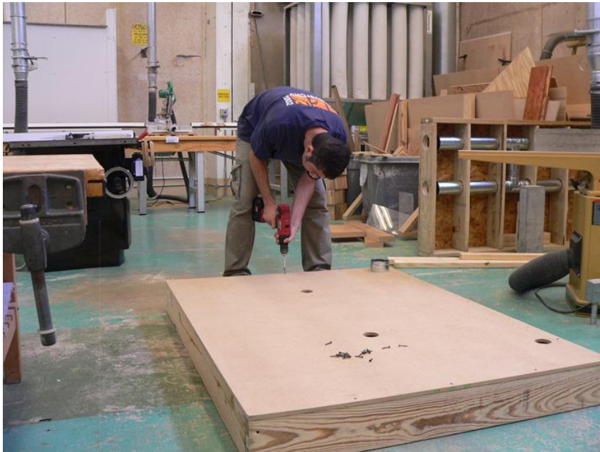
Figure A.3. Construction of the Comfort Station wall.
