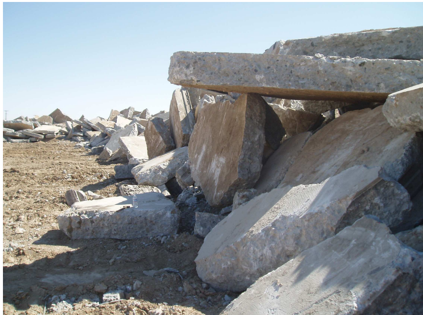
Figure 3 Stockpile of ASR Affected Concrete at Edwards AFB
