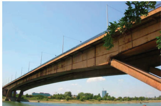
Figure 9. Major road steel bridge.
