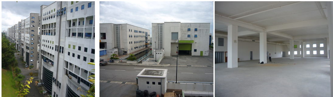
Figure 1: Plan and views of S1 complex. Lower left: stacked pairs of T2000; Lower mid: levels 5&6 of T3000; Lower right: interior of T2000 lower level
