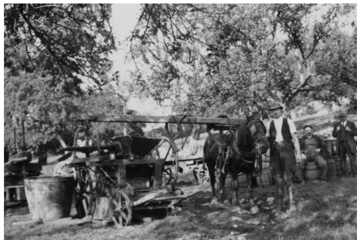
Horse-driven itinerant cider mill.
