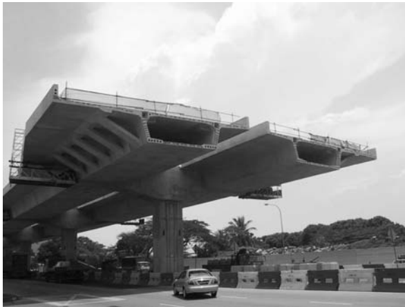
Figure 9 PPSE under construction
