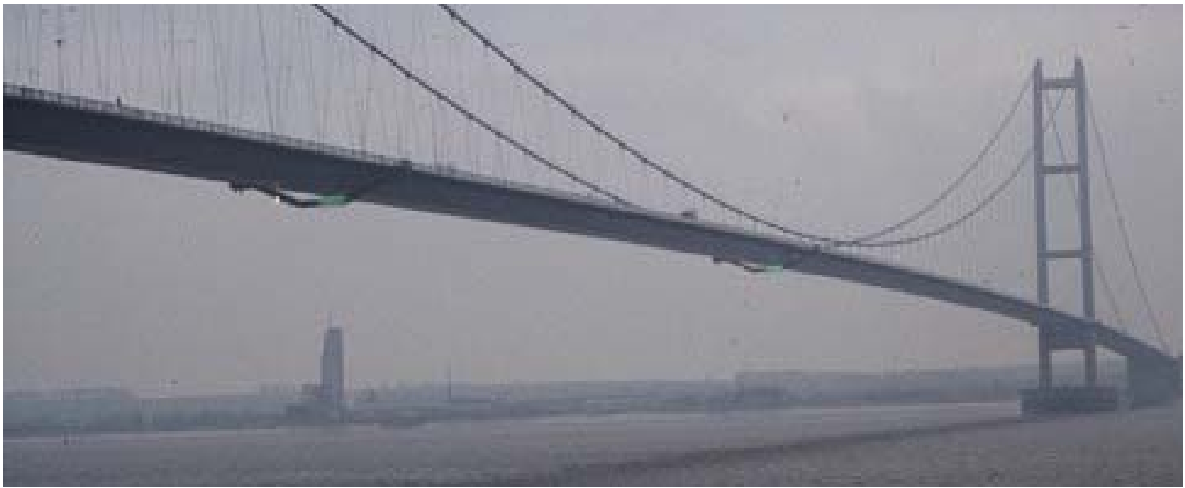
Figure 1 Humber Bridge midspan with targets for optical deflection tracking
