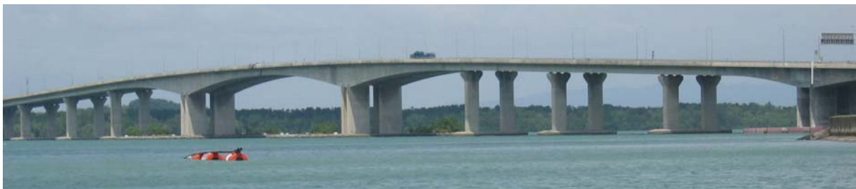
Figure 3 Second Link bridge: instrumented section at extreme right
