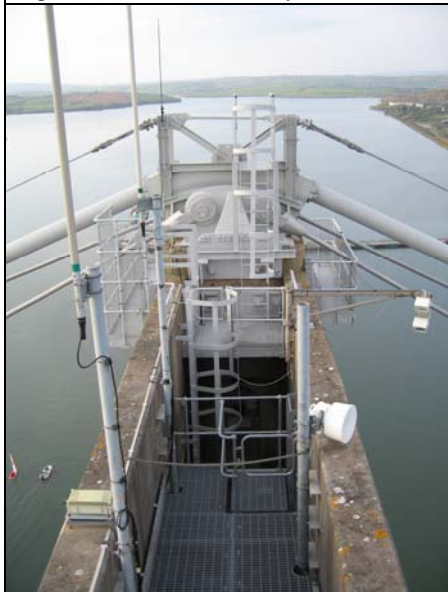
Figure 11 Saddle and stay anchorage points on Plymouth tower
