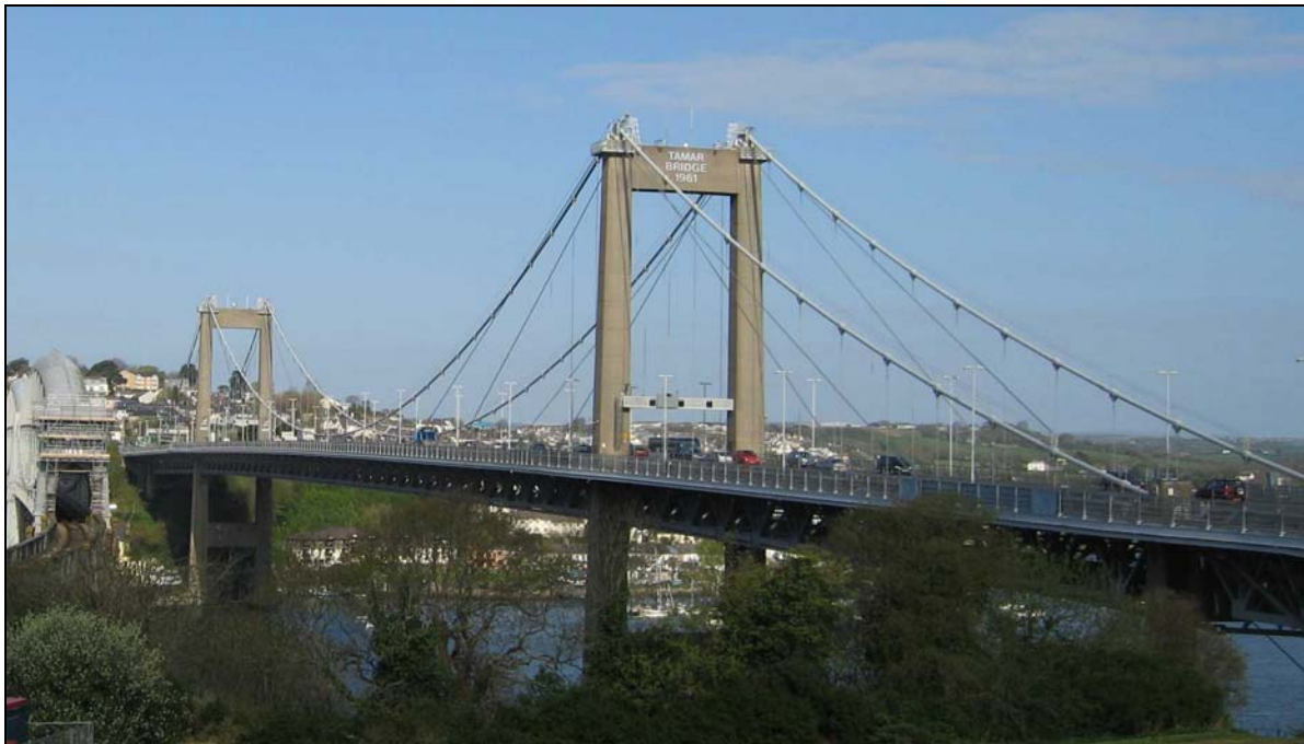
Figure 1 Tamar Bridge, Plymouth, UK
