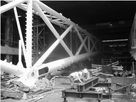
Figure 3 Arch bridge: steel frame during construction
