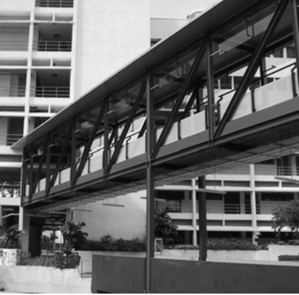
Figure 5 Walkway, with cantilevered end to left
