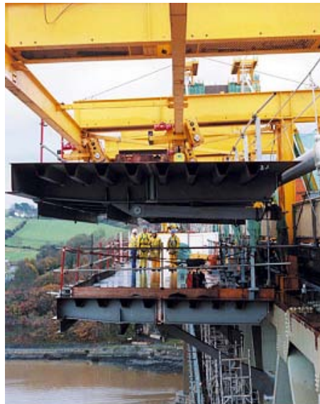
Figure 5: Installing cantilever
