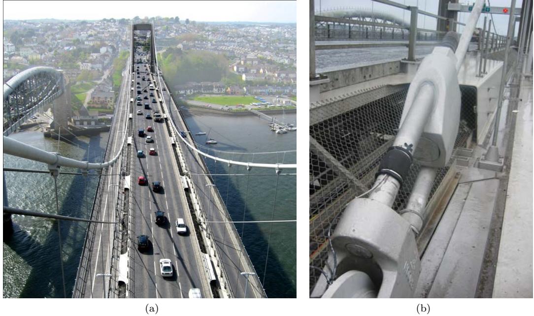
Figure 9: Shear boxes shown behind the hanger sockets (left) and additional stay connection at deck level with strain-gauges (right)
