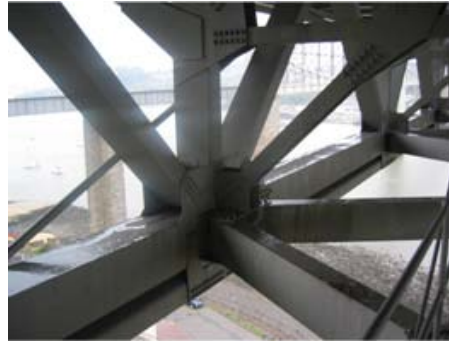
Figure 3: Deck truss and additional longitudinal girder
