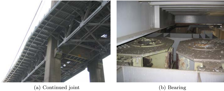
Figure 8: Bearing arrangement after upgrade
