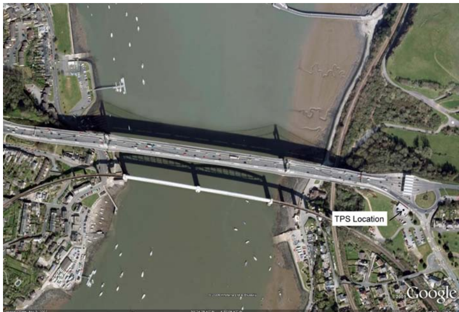
Figure 30: Birdview of Tamar Bridge
