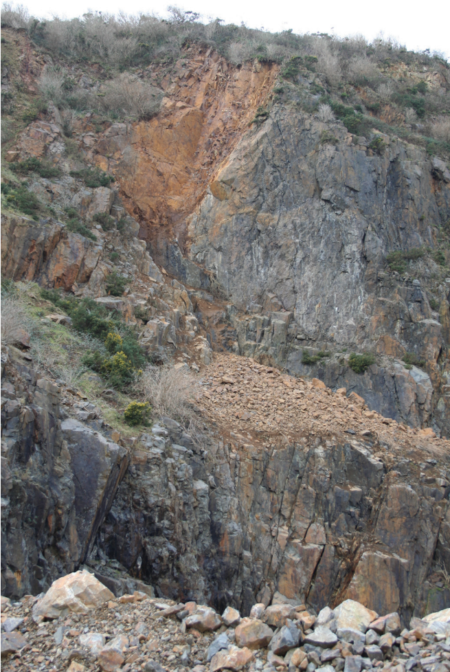
Figure 4. The January 2010 wedge failure showing the scar below the crest of the highwall and debris clogging the 45 m bench, with some spillage onto the face below. The release surfaces creating this wedge have been identified using the stereoplot in Figure 10 as Set 2 and Set 4.
