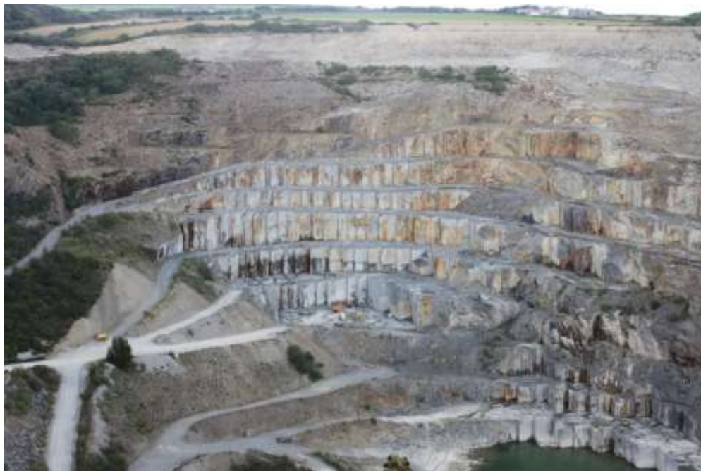
Figure 2. Photograph of the north/north-east slope taken from the south of Delabole Quarry looking north; overall slope height is approximately 150 meters, bench heights are between 4 to 10 meters
